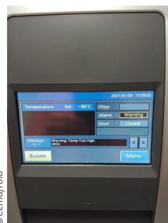
Fig. n°4 : Vaccine storage cabinet at -75^{\circ}\text{C} in the hospital and its control panel
